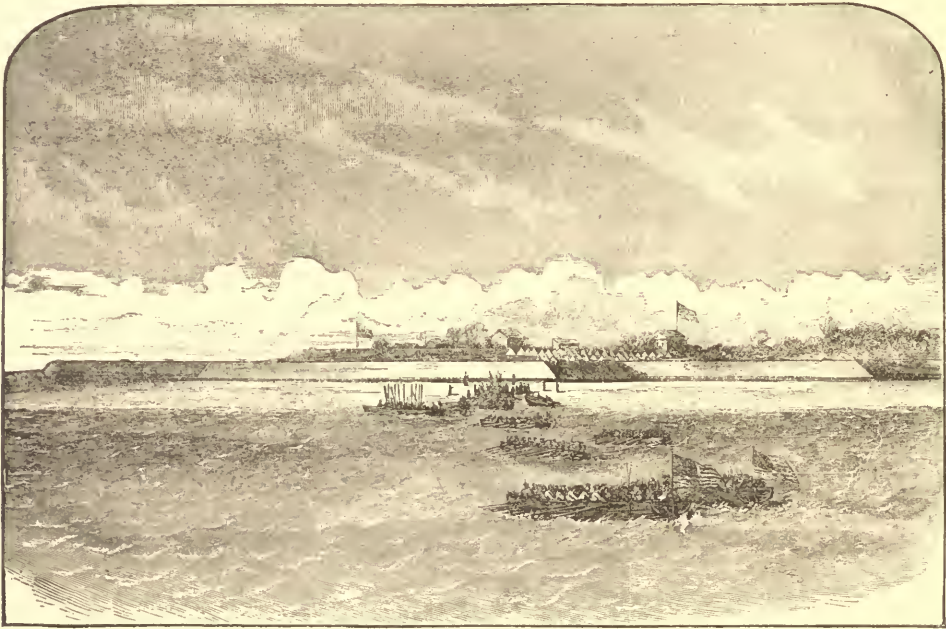
EXTERIOR OF FORT WALKER AT HILTON HEAD, MARINES LANDING.
